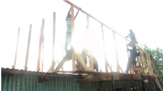
Initial stages of the construction of the semi-permanent
